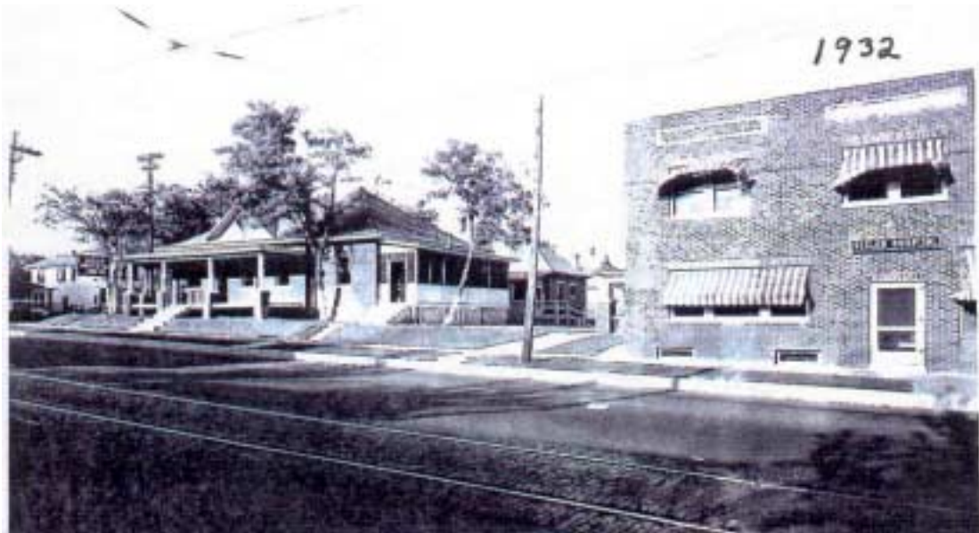
House on corner of 8 th and Elgin is The Brace Shop.. Note small sign above the door – “Sisler Hospital” and trolley tracks in the street.
